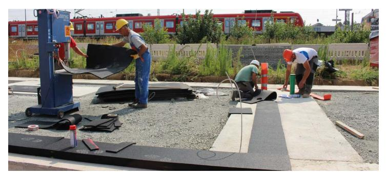
The housing precinct "Quellenpark" has successfully managed these obstacles. A 300-meter-long building complex has been built parallel to the railway track in a distance of just 14 m. Thanks to an elastic decoupling of the building's strip foundations this development is being protected against ground-borne vibration and secondary air-borne sound.
